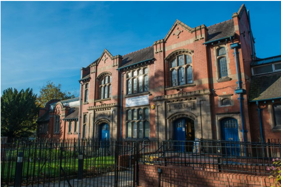
The historic council-owned Withington Baths that have been leased to the Love Withington Baths organisation since 2015.
