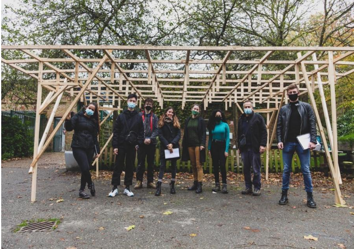
Figure 4: Teamwork building the space frame structure, 2020
