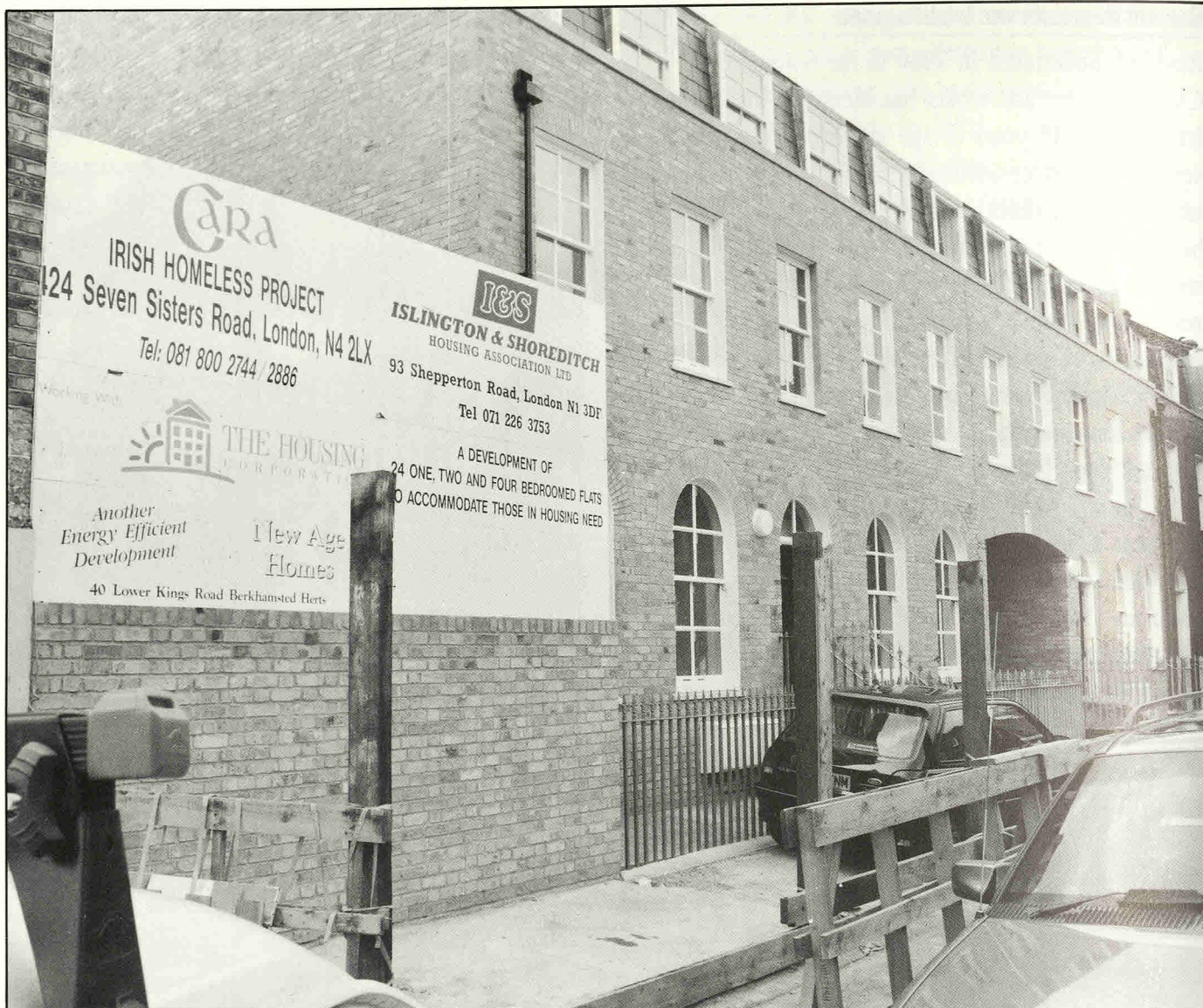
New scheme nearing completion in Islington
