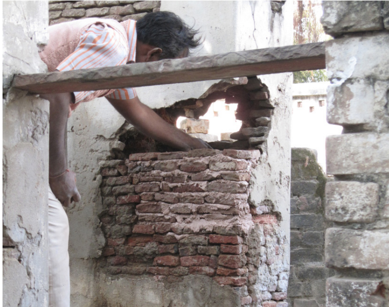
The Raj Mistry repairs the structure with reclaimed bricks
