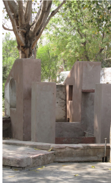
Well structure before and after repair
