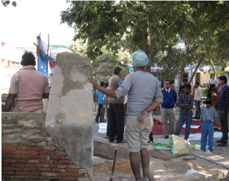
A Raj Mistry repairs the well structure
