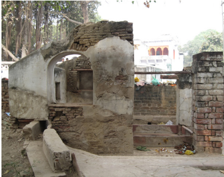
Well structure chosen for conservation repair workshop
