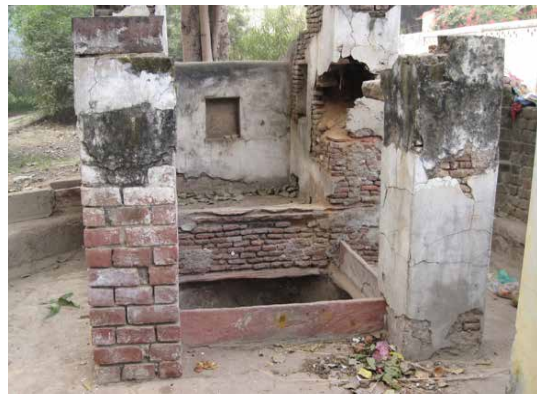
Structure before restoration
