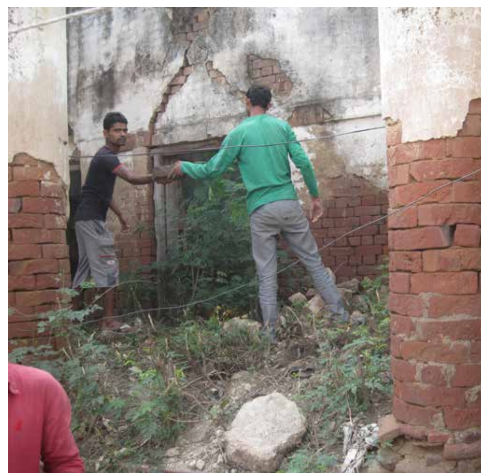
Clearing rubble from upper terrace
