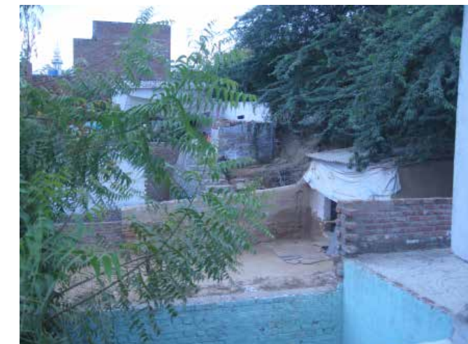
4. Cheap brick construction
