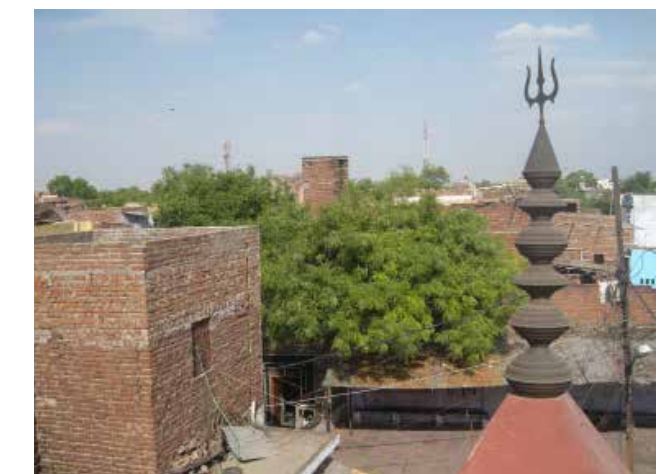
Replaced every 300 years
