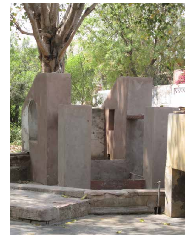
Structure four months after workshop
