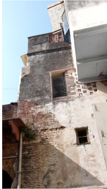
Recent, unregulated additions to buildings over 100 years old
