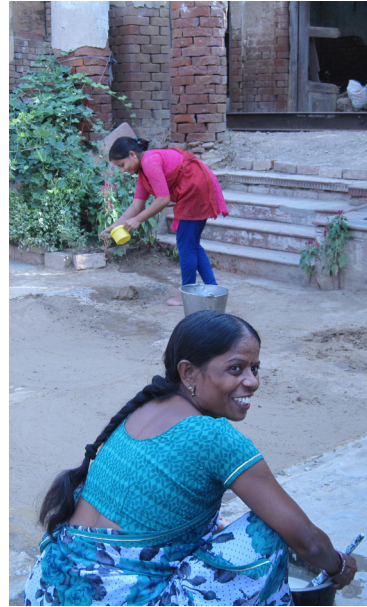
Using rubble from Level 01 to create a new floor at Level 00 at the Buksh House (left) and laying a new earth floor (right)
