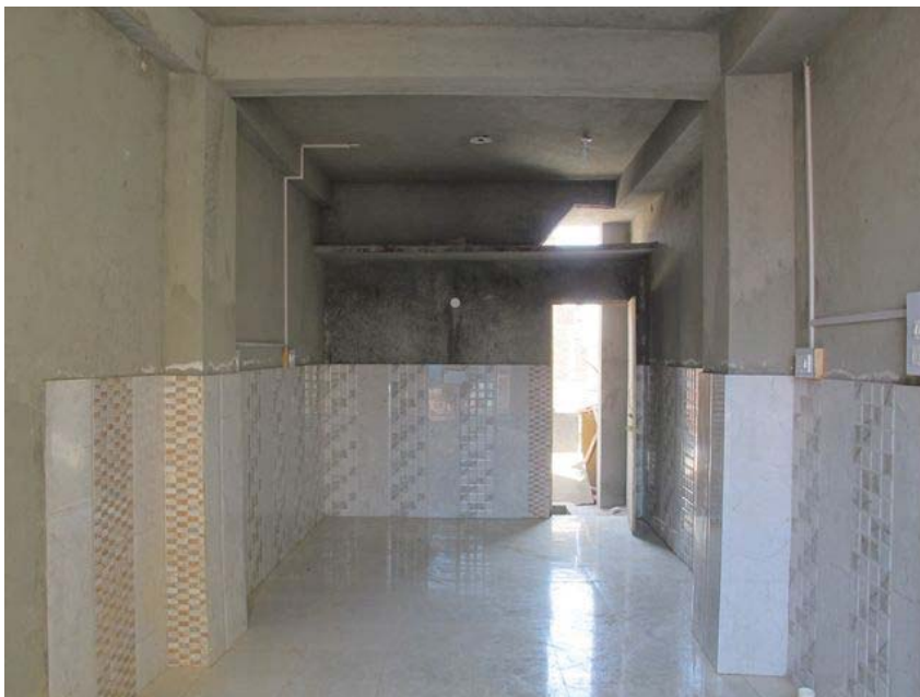
Image 3.2.6 INTERIOR SHOT OF CORE HOUSE. This is a photograph of the first floor (ground plus one) which will house the water treatment plant. The room has been tiled to not only keep the room clean (important both practically and in terms of public image) but also to have a surface which can manage water spillage. Tiling is also perceived as the most premium finish for a house.
