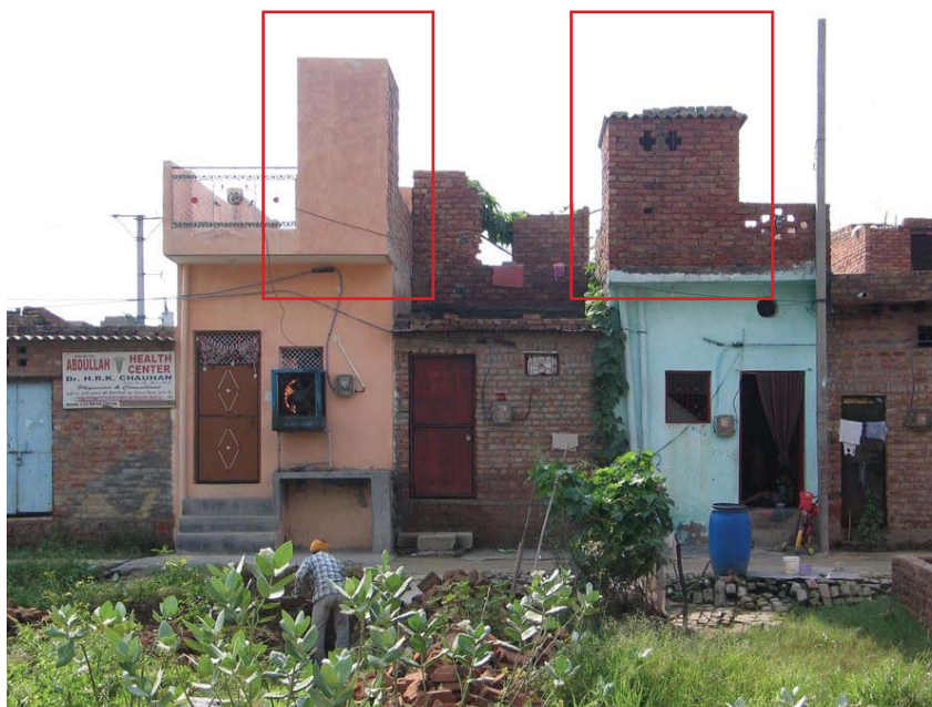
Image 3.5.5 (top) and 3.5.6 (bottom). HALF INCREMENTS. Both houses are pucca with a half increment. The families have built a toilet structure on the first floor. A black water waste pipe can be seen to the front left of the house in both cases. The house on the right has lost half its living space on the ground floor to a shop so another room has been built on the first floor. The house to the left is occupied by one family so all living takes place at ground level. In both cases all washing and water-based activities happen on the first floor open to air space.
