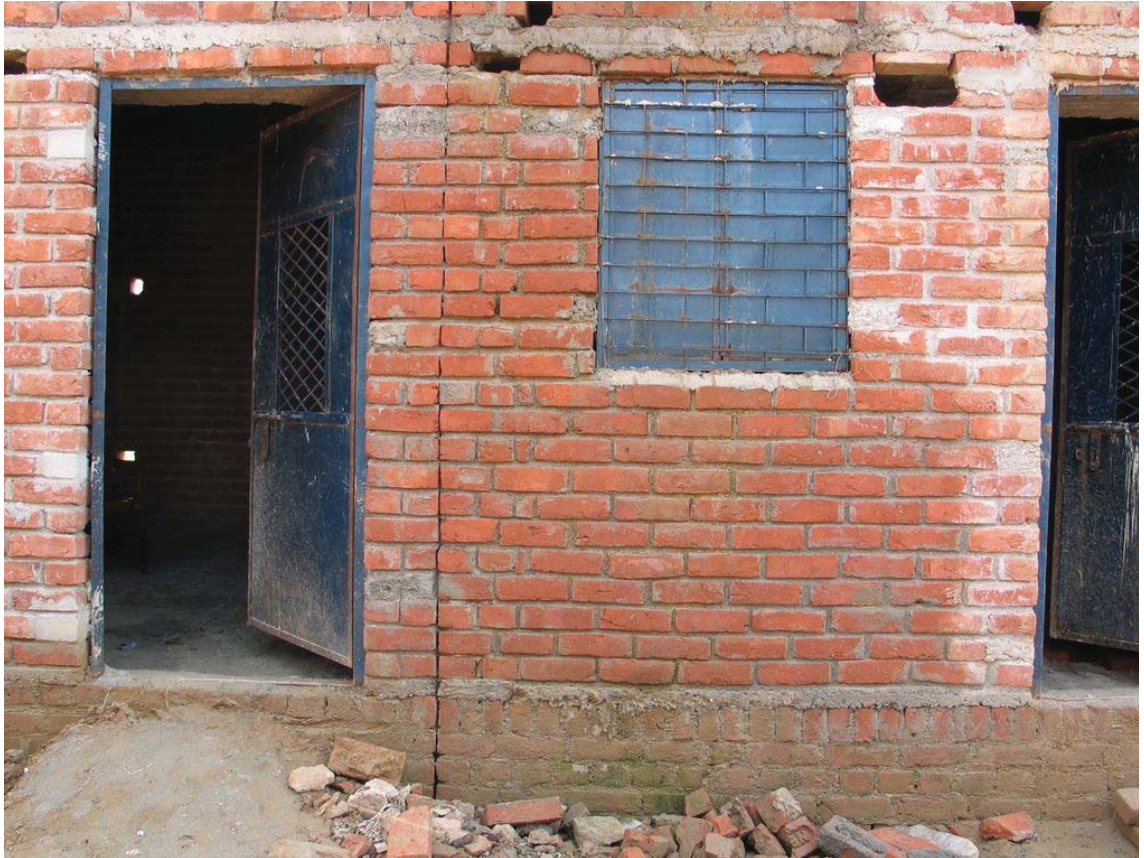
Image 3.2.1 DETACHED HOUSING. This image clearly shows the very small gaps between houses.
