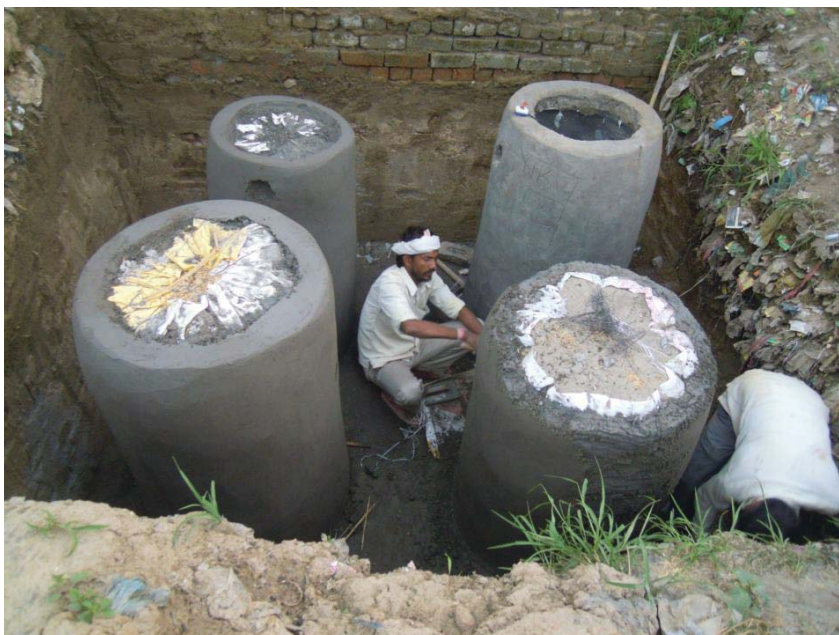
Image 3.1.13 SELF INITIATED FERROCEMENT PROJECT. Rainwater harvesting and groundwater recharging.
