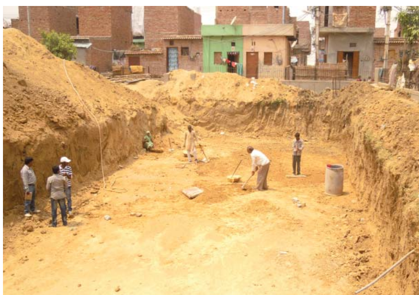
Image 3.3.8. EXCAVATION WORK FOR SEPTIC TANK AND UP-FLOW FILTER. The septic tank services up to 350 households, with an average of six people per household, with a two year maintenance plan.
