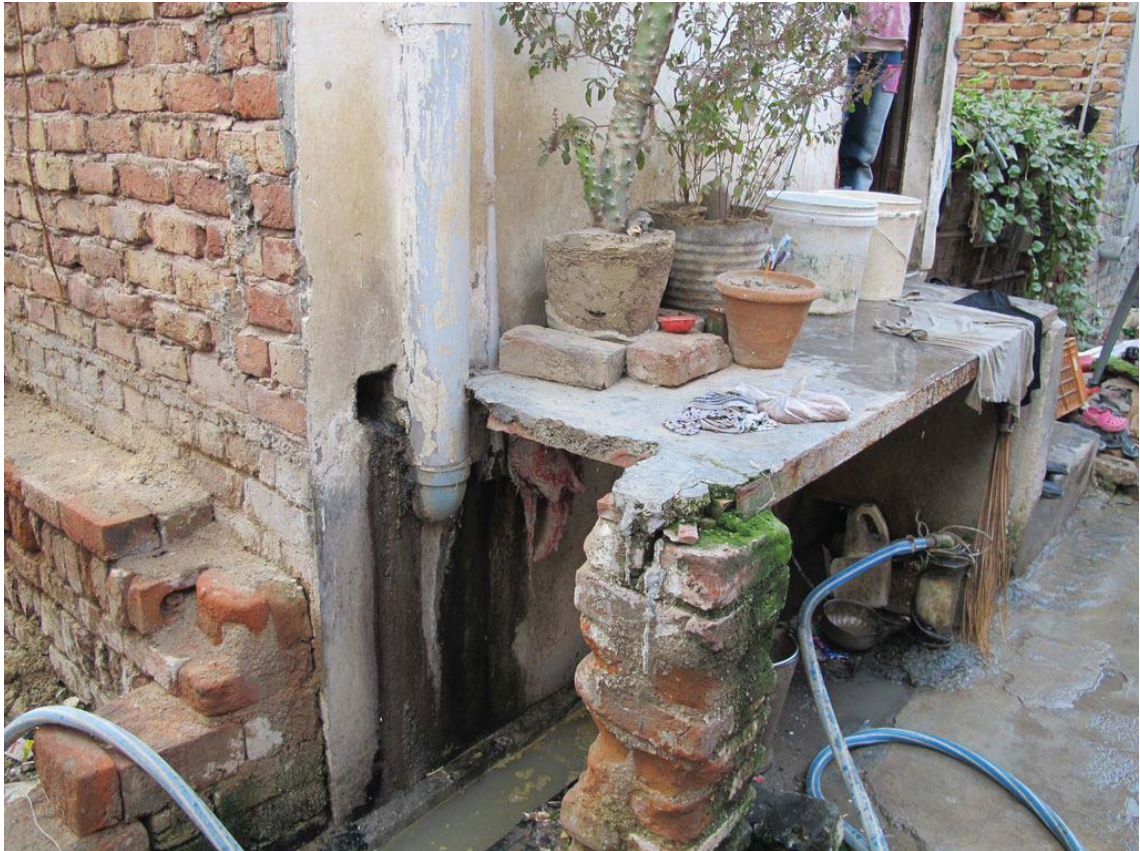
Image 3.3.1 TYPICAL OUTLET RELEASING EFFLUENT INTO OPEN DRAINS. The tanks often overflow into what are incomplete and blocked open drains intended to move greywater leaving exposed sewage to stagnate and percolate into the ground. Not all houses let their tanks overflow and will get the
