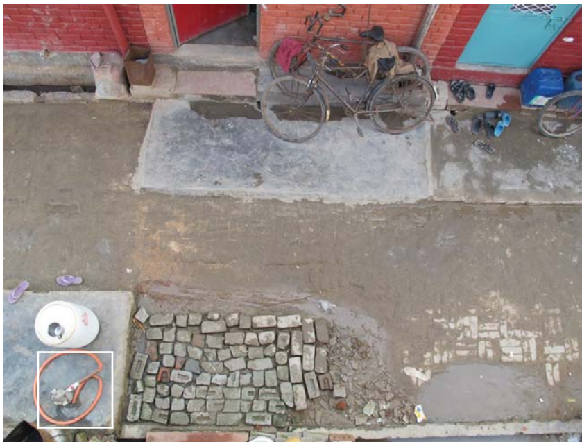
Image 3.4.2 INSTALLED BOREWELL. Small scale changes occur following the arrival of the borewell as the urban fabric accommodates this. The borewell is placed on a plinth which is to secure the borewell but is also part of a legitimizing process. The area surrounding the borewell is roughly paved with broken left over bricks which helps drain away the water which spills to the ground as people fill up their buckets. What might look haphazard is a sophisticated low cost response to infrastructure.
