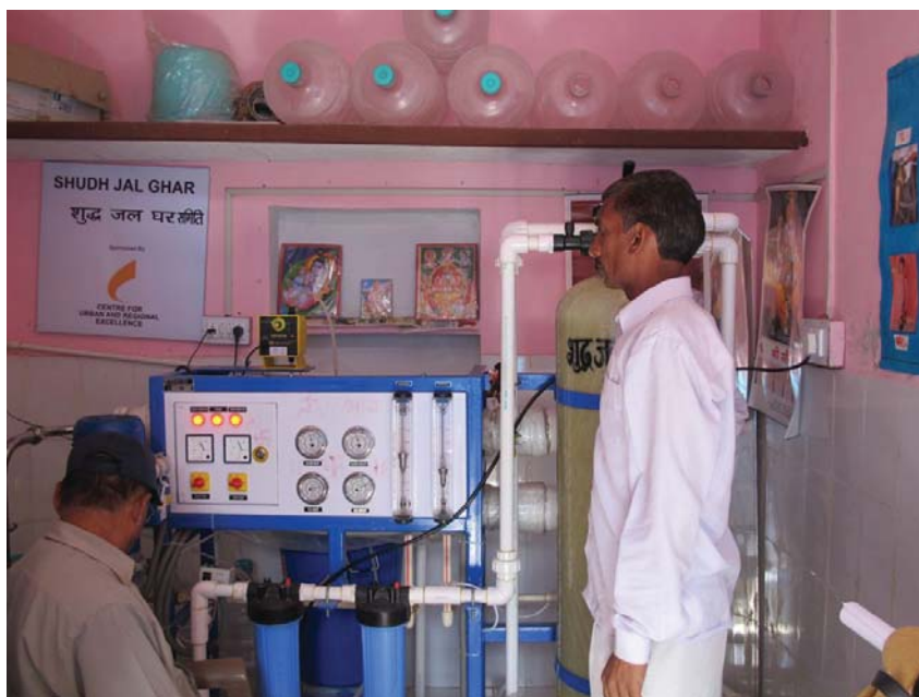
Image 3.4.7 WATER KIOSK AND FILTRATION SYSTEM. This is an internal shot of the Water Kiosk showing the filtration plant.
