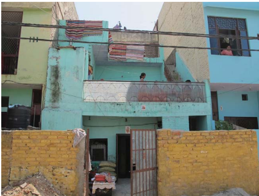
Image 3.6.6 HORIZONTAL INCREMENTS. The Singh family moved to Kalyanpuri in 1979 and purchased the second, neighbouring, plot not long afterwards. They are currently renting another apartment and refurbishing the entire ground floor to accommodate a new bride who has married into the family. They are adding another kitchen and are looking at adding another floor in the future when their younger son marries.
