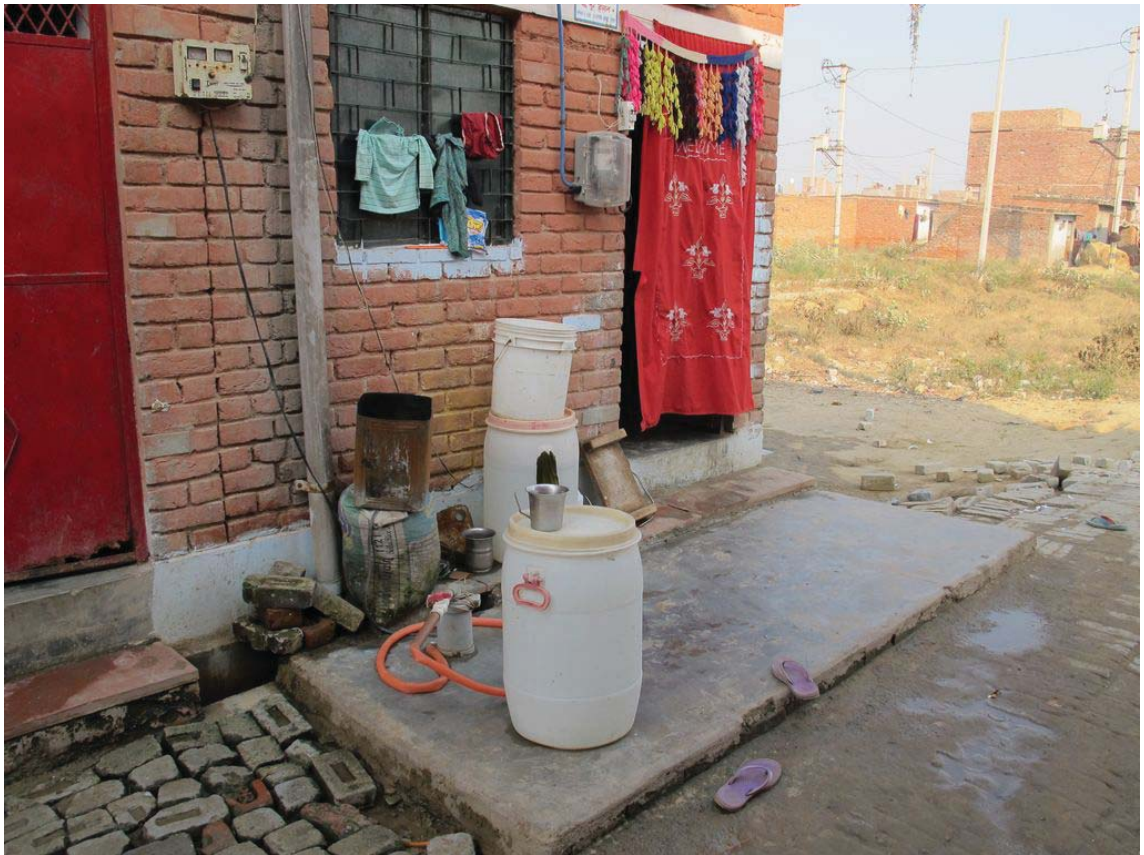
Image 3.4.3 INSTALLED BOREWELL AND PLINTH.
