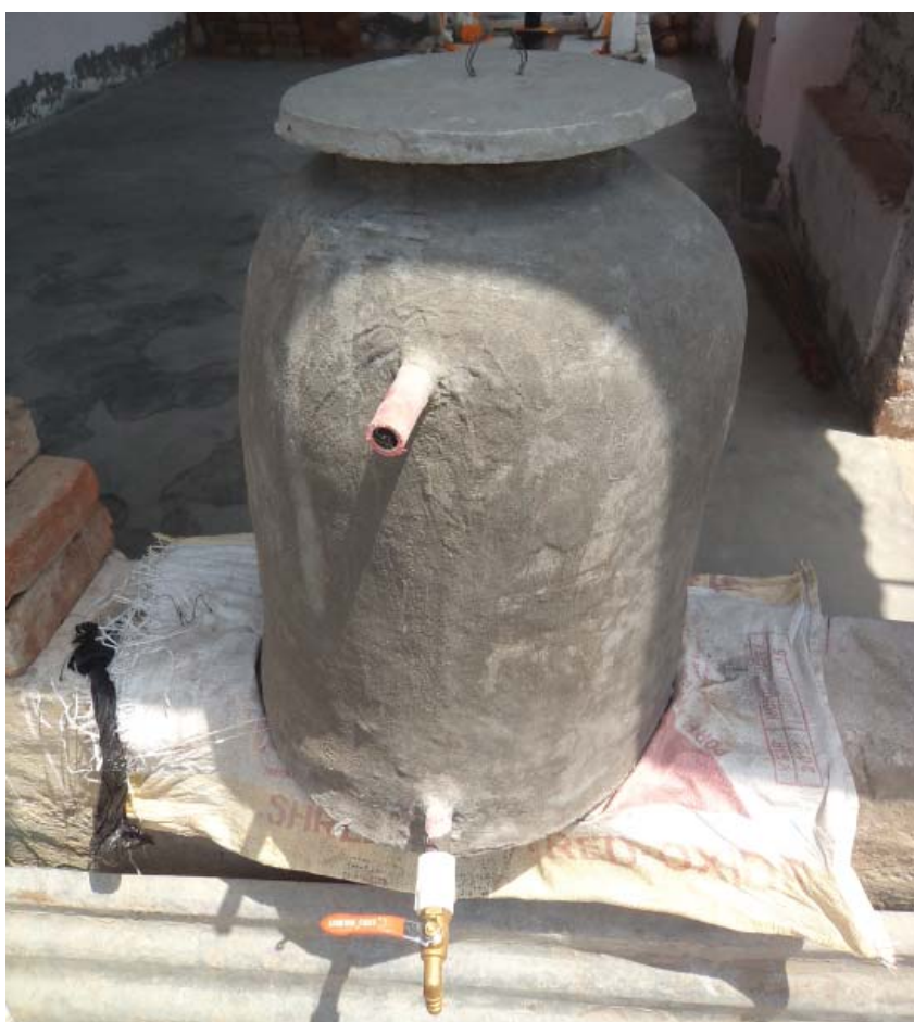
Image 3.1.10 FERROCEMENT RAINWATER HARVESTING TANK. The workshop was run over the course of one afternoon which limited the scope of what could be built, ultimately limiting the size of the tank. Unlike the first cycle, this tank used a formwork: readily available hessian sacks used to transport cement. This principally determined the size and shape of the tank: the sack was filled with sand and then the wire mesh and mortar were formed around the shape. Once the mortar had set, the sand was removed through the top leaving a thin shelled jar. For the inlet and outlet small plastic pipes were inserted and cast into the tank, allowing for simple additions such as a nozzle to be affixed later.
