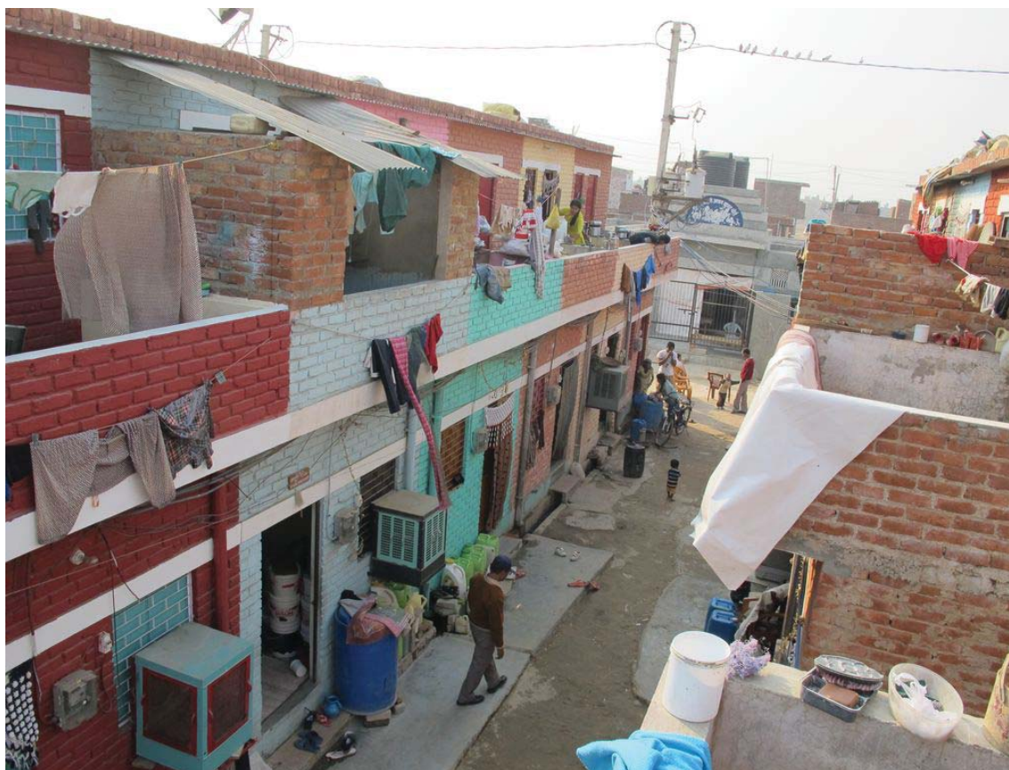
Figure 3.4.4 'AKT' HOUSES. The simple brick and concrete houses were designed such that the residents themselves could alter and add-on with ease. For example, rather than have a pucca reinforced concrete roof
