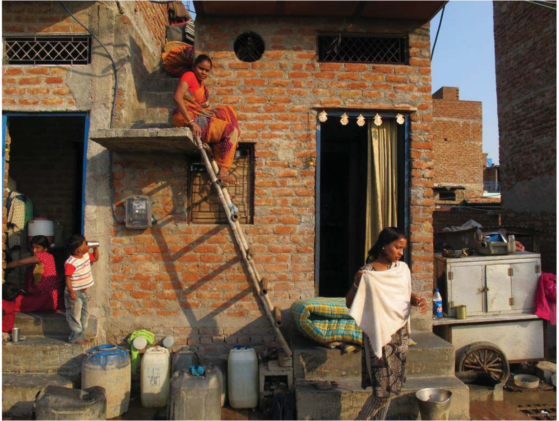
Image 3.1.4 BAMBOO STEPS. Rather than build a concrete staircase this family is using a bamboo step ladder to access the roof. Bima, who owns the house, described this as an incremental addition that will later become more 'permanent' when another floor is added which would ideally also have a toilet; whereupon they will get rid of the bamboo ladder and replace it with a set of reinforced concrete steps.
