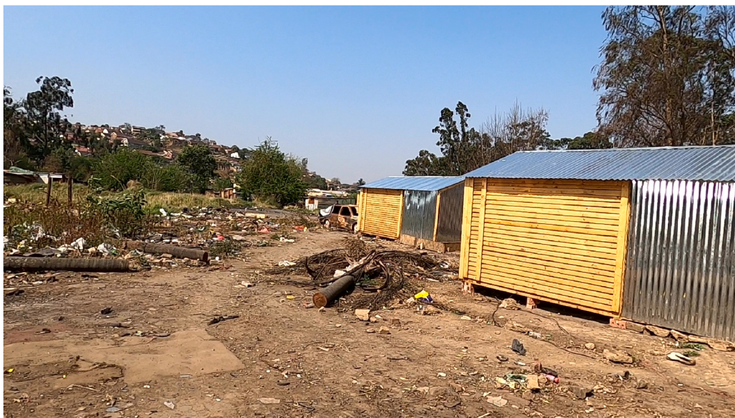
Fig. 5. Low-lying ground and poor surface drainage adjacent to dwellings rebuilt after a fire in Khan Road; unlike the original self-built shacks, these units are raised above ground level.
