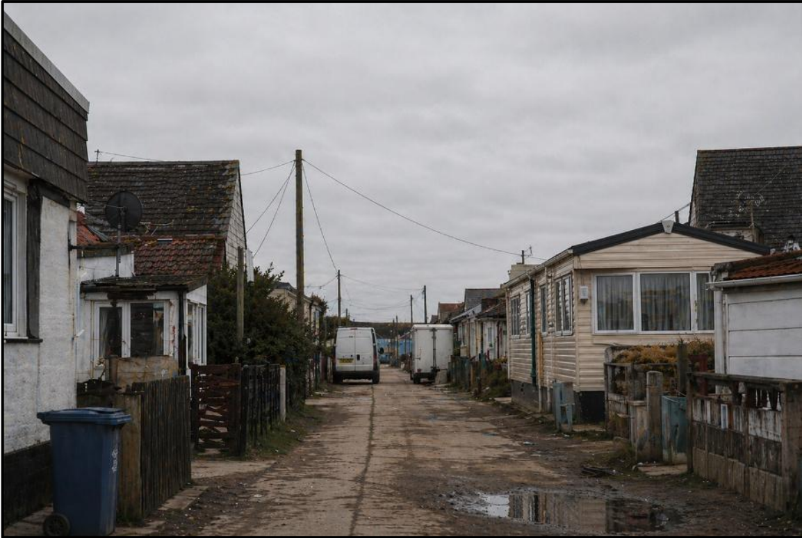
Photograph to show poorly serviced street in the UK (source: Centre for Security Research and Studies).
