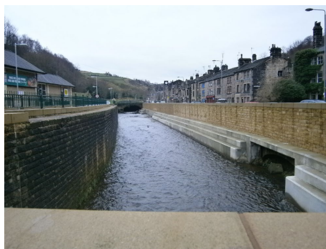
FIGURE 4 | A flood wall part of the Todmorden scheme. Source: Authors.
