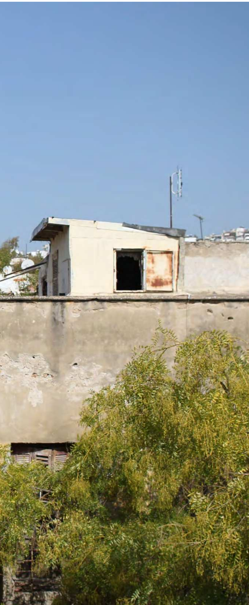
Left Rooftop in Prosfygika (Jameson Goring)
