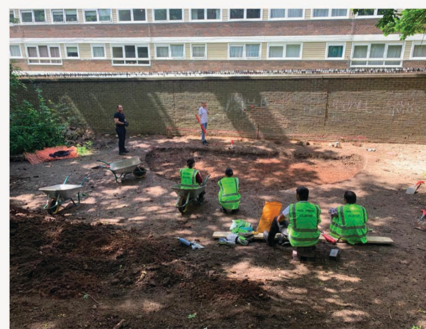
FIG26 - GROUND WORK - 5 JULY 2021
