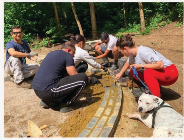
FIG.34 - START OF THE BRICK STAGE
