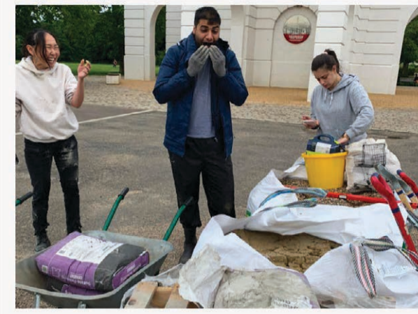
FIG.32 - TEAM UNLOADING MATERIALS DELIVERY
