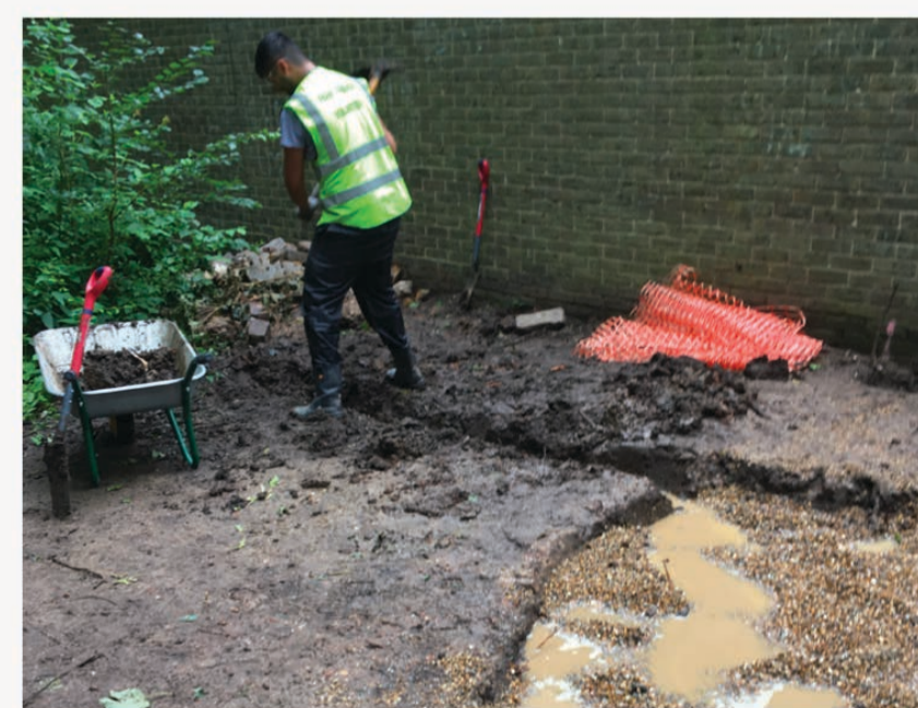
FIG27 - GROUND WORK - 7 JULY 2021
