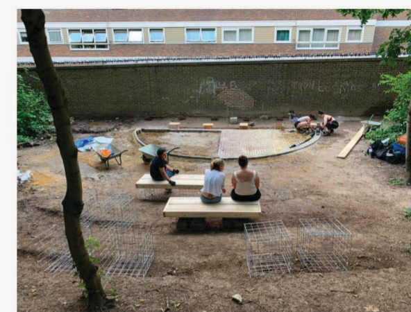
FIG.43 - THE BRICK STAGE WORK
