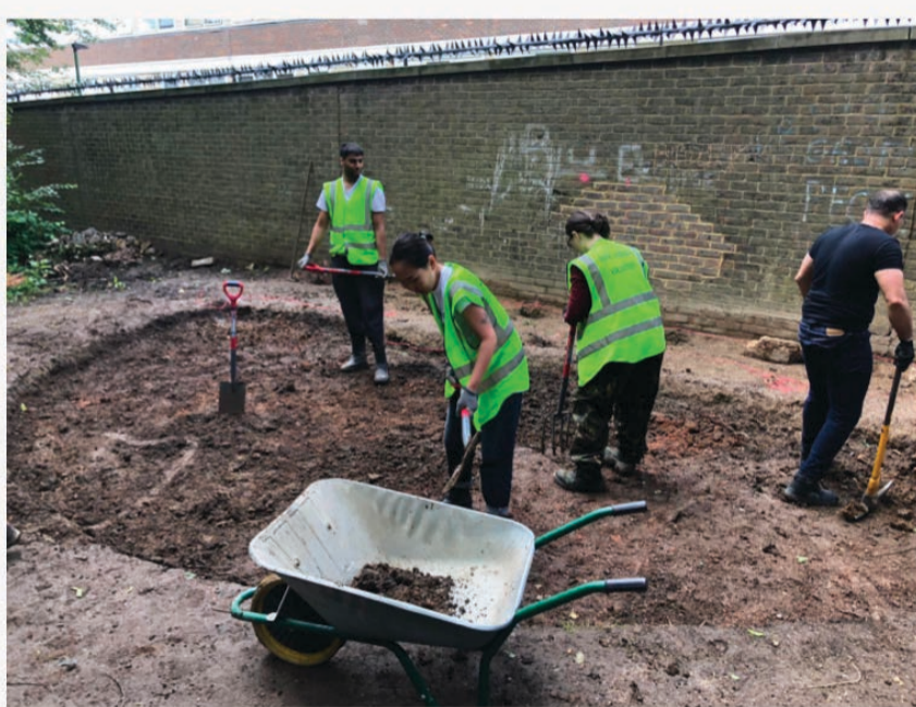
FIG25 - GROUND WORK - 5 JULY 2021
