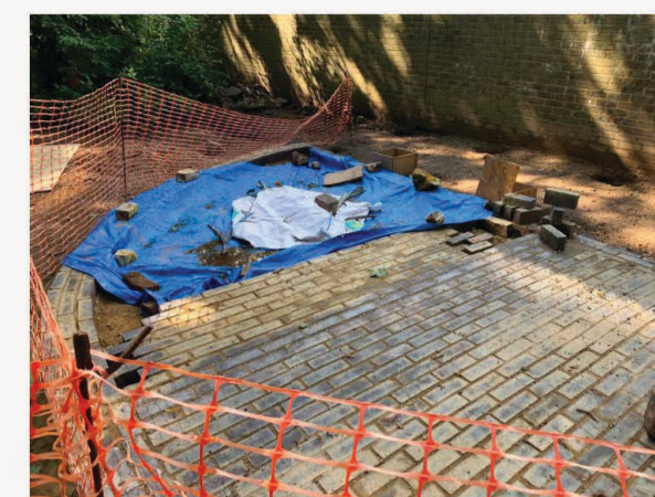
FIG.44 - UNWRAPPING THE STAGE IN THE MORNING
