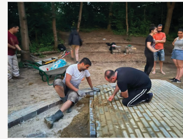
FIG.39 - THE BRICK STAGE WORK
