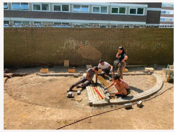
FIG.37 - THE BRICK STAGE WORK
