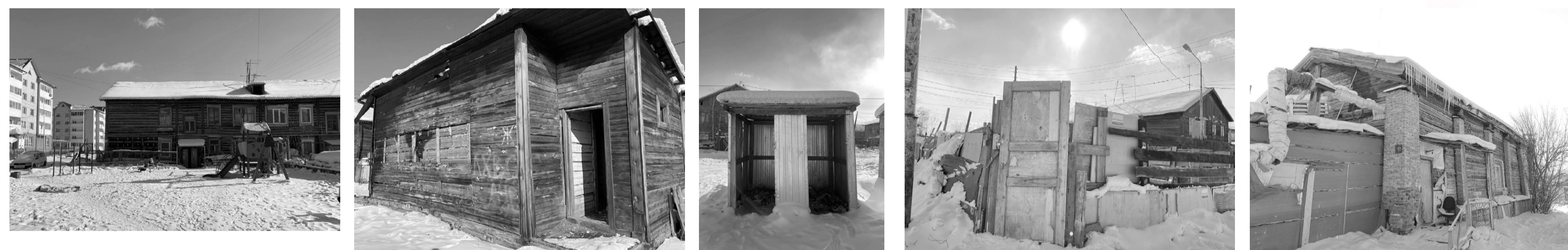
Site photos 17th district
