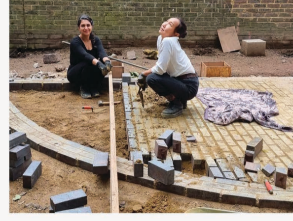
FIG.45 - THE BRICK STAGE WORK
