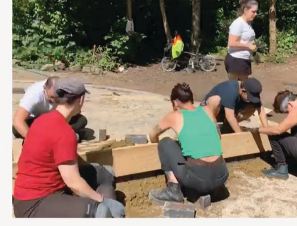
FIG.45 - THE BRICK STAGE WORK
