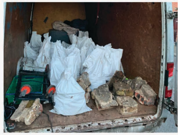
FIG.33 - TEAM UNLOADING MATERIALS DELIVERY
