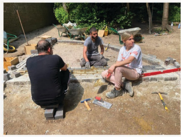
FIG.36 - THE BRICK STAGE WORK
