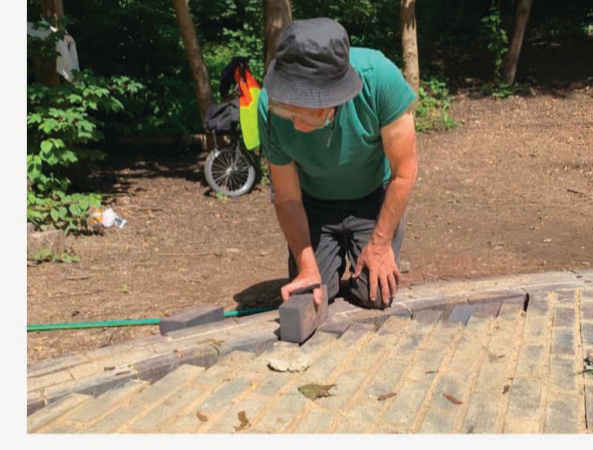
FIG.47 - MAURICE CUTTING THE EDGE BRICK
