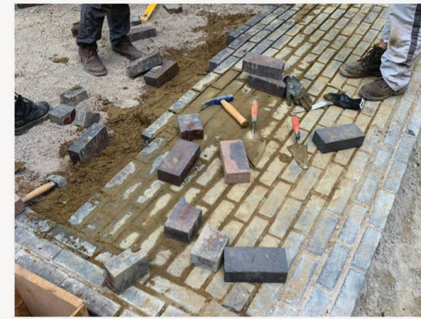
FIG.38 - THE BRICK STAGE WORK
