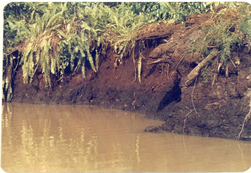
PLATE 10. In some localities, river bank erosion has cut into and exposed the peat deposit.
