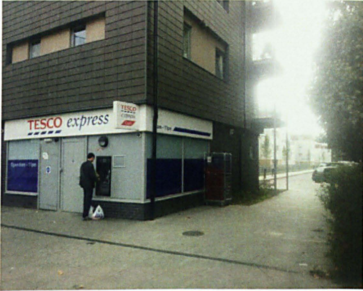
Fig. 52 Location 1: the western end of the Tesco Express on Bow Road, adjacent to the cash-point, where there is pedestrian access to and from British Street (photo by author 24 th Sept 2011).
