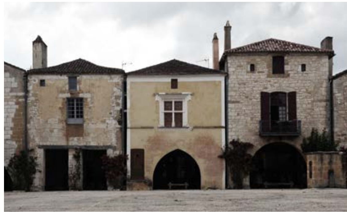
9. Different characters of façades of houses on the west side of the Place des Cornières. Photo: David Jones, May 2016.
