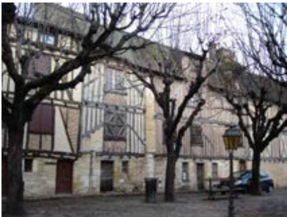
19. Timber frame and infill construction, Bergerac, November 2009.
