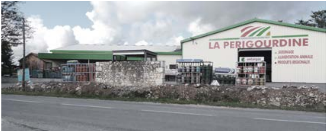
49. Wall remnant and cooperative industrial shed on the road to Beaumont, September 2013.
