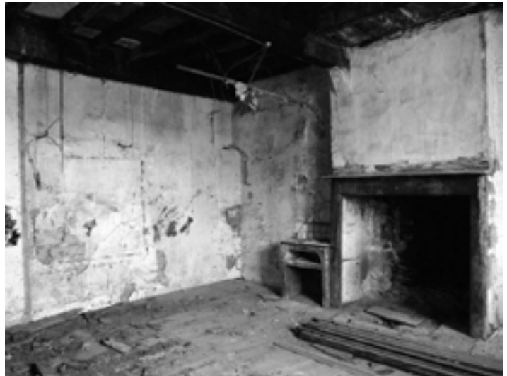
67. First floor room in a derelict house on the north side of the Place des Cornières, November 2009.
