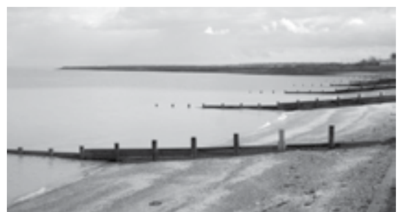
46. Coastal groynes, Dawlish Warren, Devon. Photo: N Chadwick.
