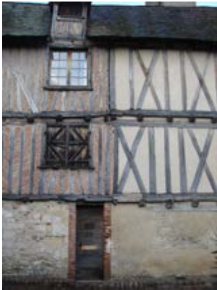
18. Timber frame and infill construction, Bergerac, November 2009.
