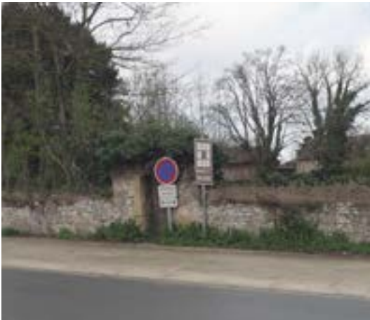
35. Overgrown walled garden in the grid extension north of the bastide, April 2010.
