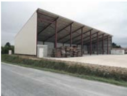
50. Large open-sided shed north of the road to Beaumont, September 2013.
