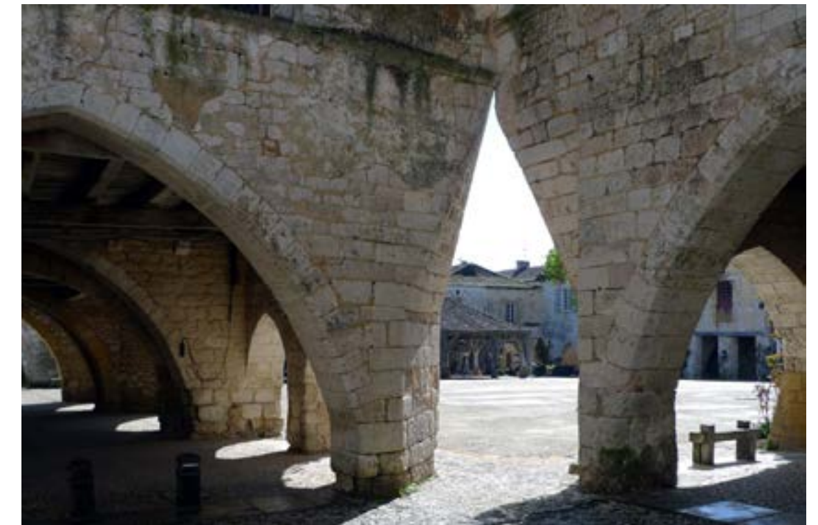
20. Higher arched opening leading diagonally into the Place des Cornières. November 2009.
