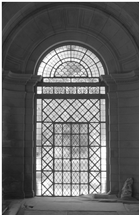
Figure 2. Original window in Millbank Foyer
