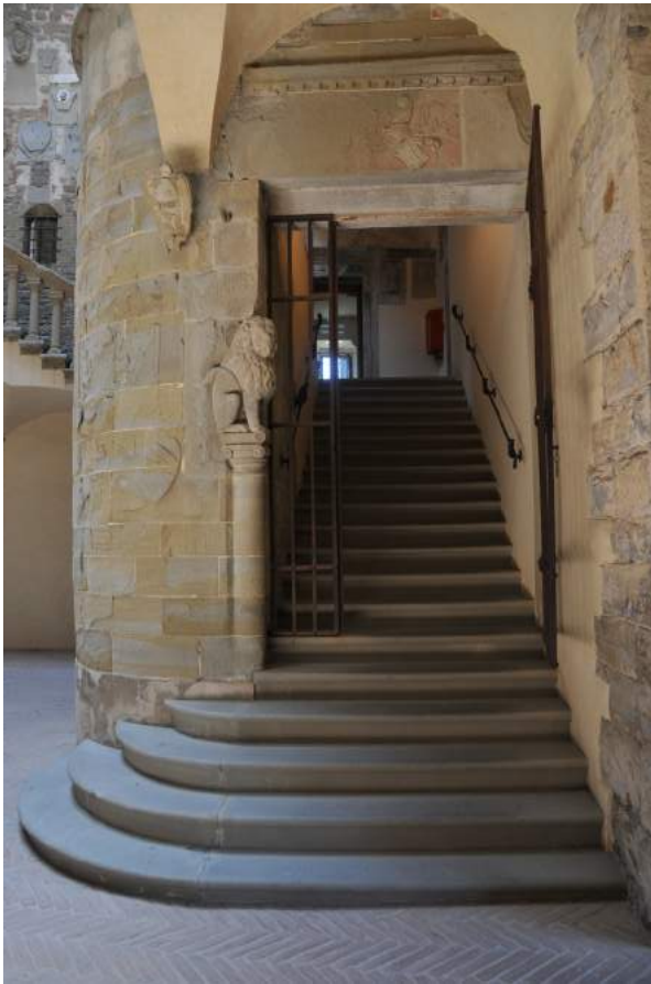
Figure 5.11. Poppi Main Stair up to First Floor
