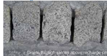
Drains through stones above recharge pit
