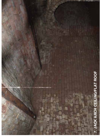
7. JACK ARCH CEILING/FLAT ROOF (view above)
