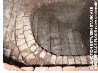
6. JUNCTION BETWEEN STAIRCASE AND TERRACE FLOOR
